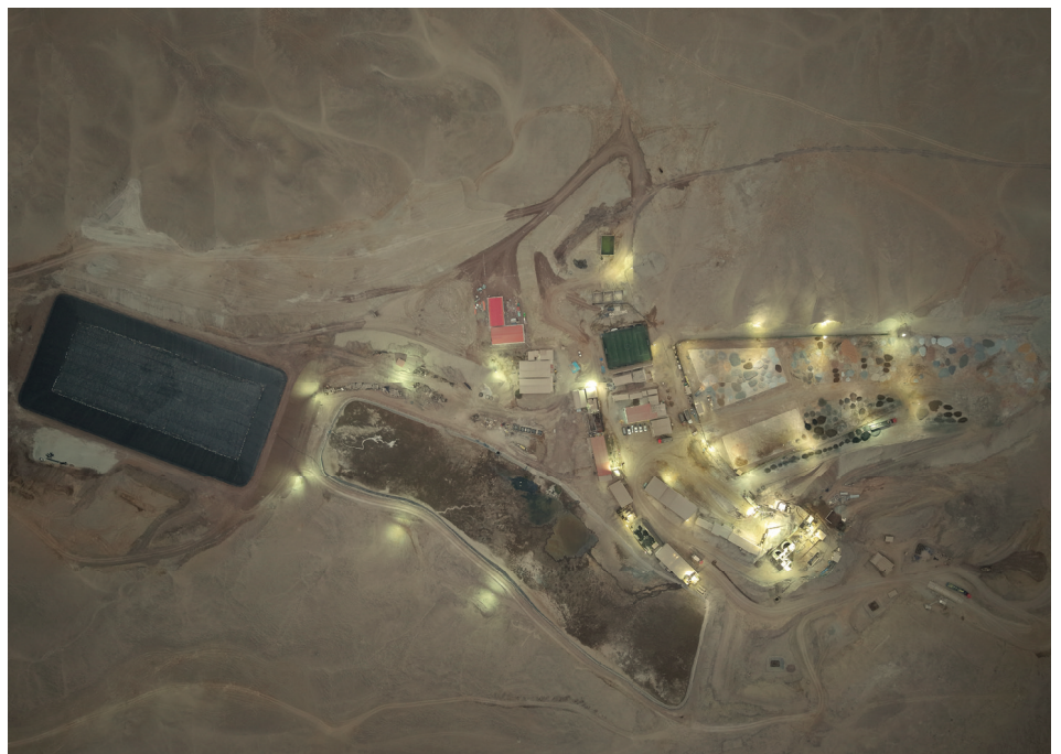
Aerial view of processing plant facilities in Victoria.
