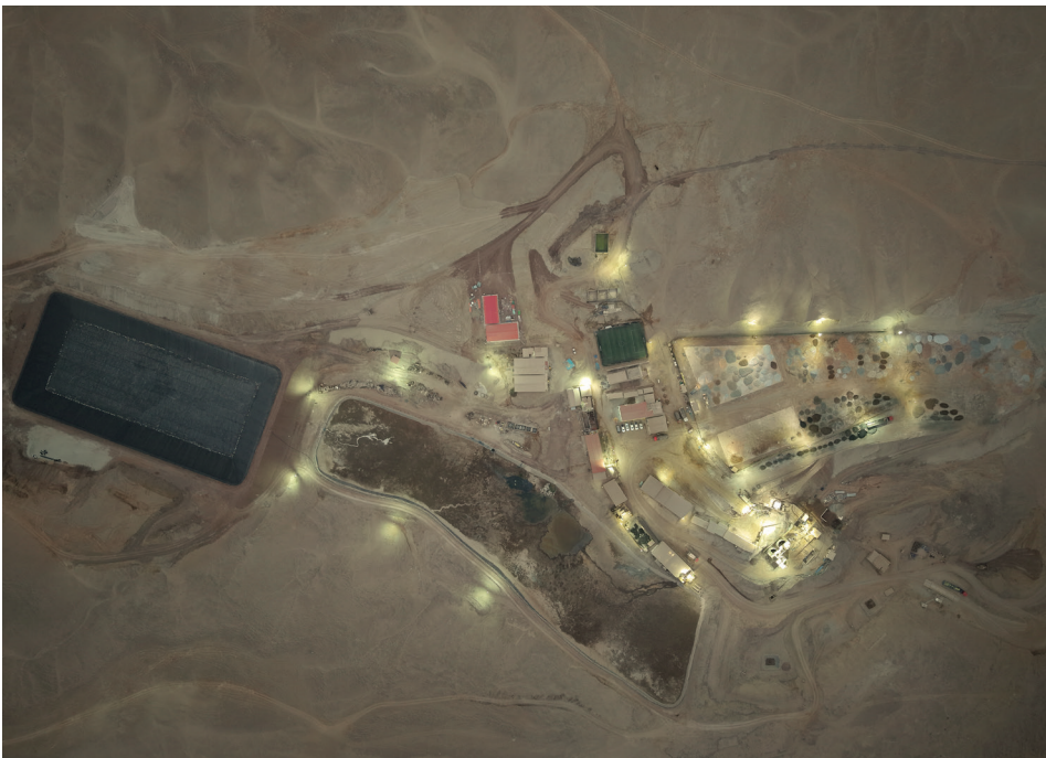
Aerial view of processing plant facilities in Victoria.
